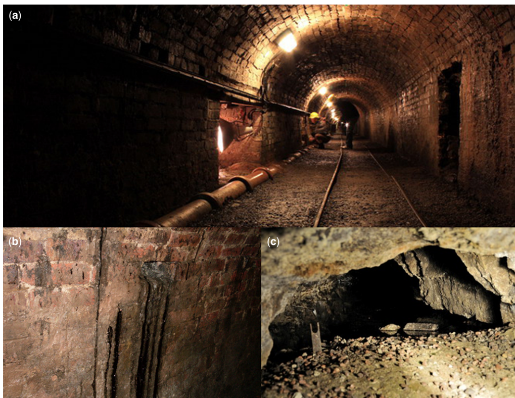
Fig. 3. The Coalport Tar Tunnel, Ironbridge, Shropshire. (a) The Tar Tunnel with a drainage pipe on the left and wells cut into the tunnel walls. (b) Bitumen oozing out of the brick-lined walls. (c) A pool of bitumen in one of the wells ( http://geotopoi.wordpress.com/2012/09/13/coalport-tar-tunnel/ ).
