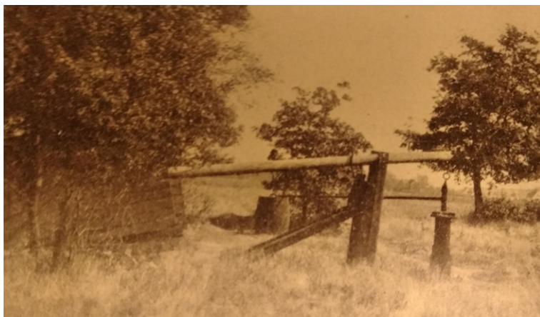
Fig. 5. The first commercially productive oil well drilled in the Wietze Field, Hannover, Germany. Drilled by the Hannoverian government in 1859, the well yielded a small amount of oil at a depth of about 100 m. Until the 1930s, it was occasionally pumped by hand. From Rinehart (1930) .
