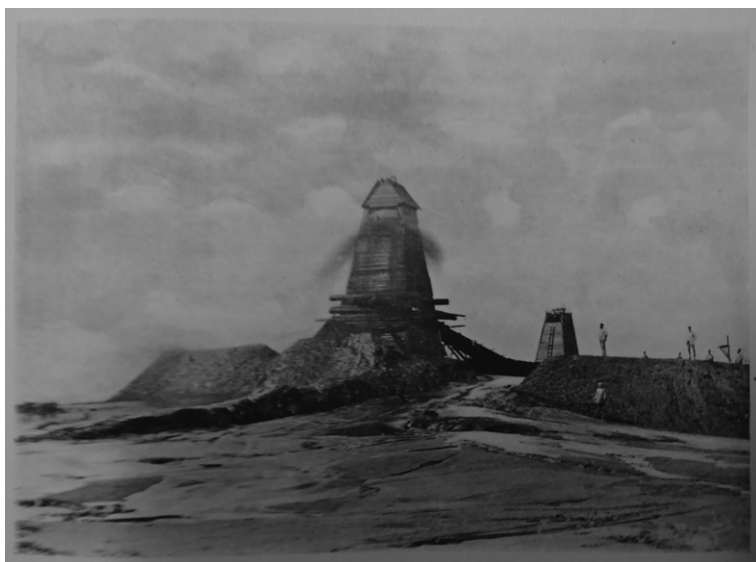
Fig. 6. A Baku ‘spouter’. The derrick is almost buried in sand ejected from the well (from Beeby-Thompson 1904 ).
