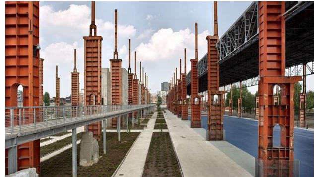
Figure 1. Ex- strippaggio factory, Teksid area
