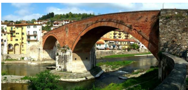
Figure 1 - View from the right side of the bridge, current state.
