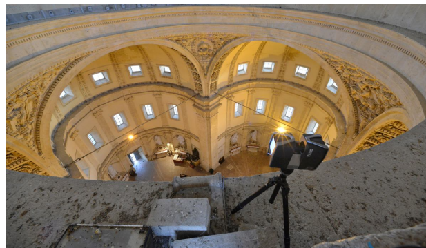
Figure 10. Internal scan from the dome base
